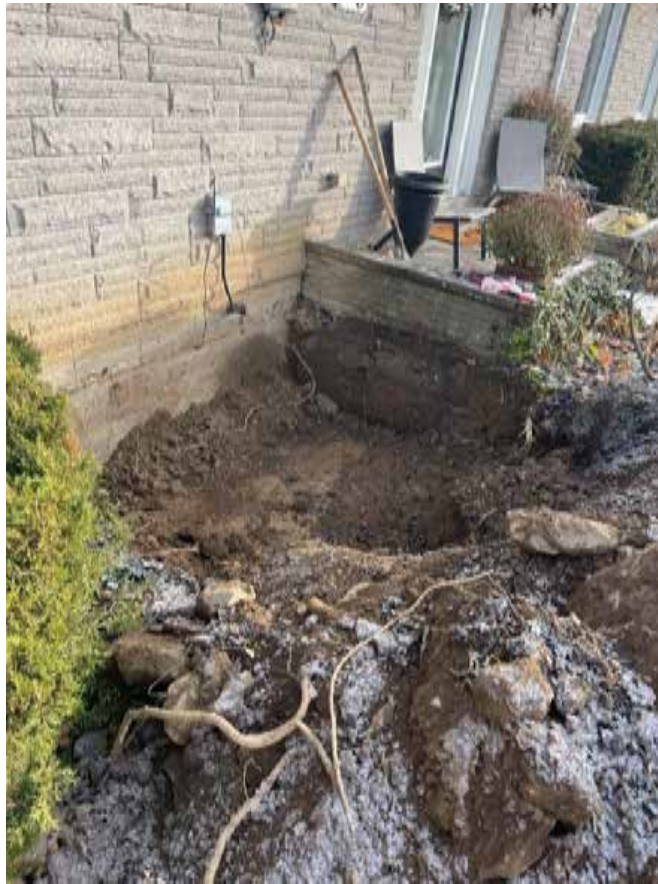
PHOTO 4 – NORTHEAST VIEW EXCAVATION AFTER TANK REMOVAL.
