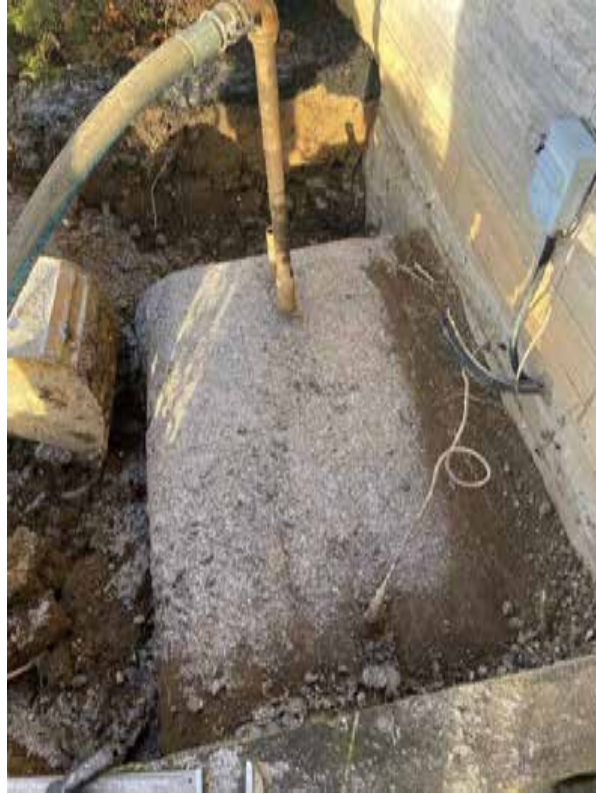
PHOTO 1 – NORTHWEST FACING VIEW OF THE TANK NEST PRIOR TO TANK REMOVAL.
