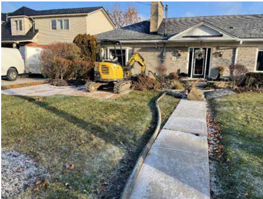
PHOTO 2 – NORTH FACING VIEW DURING EXCAVATING.
