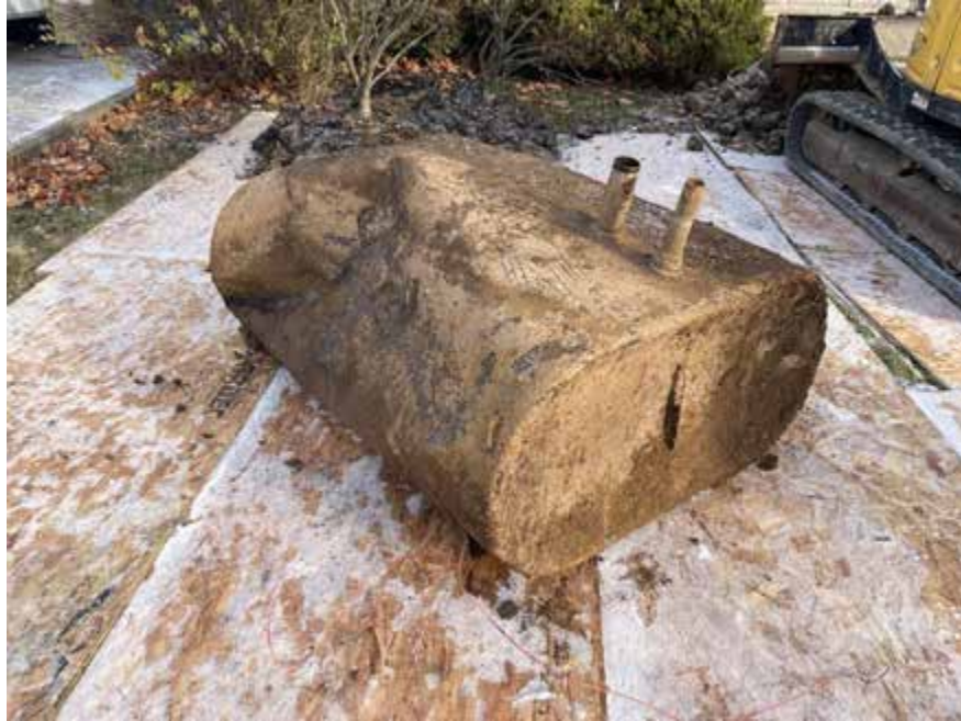
PHOTO 3 – VIEW OF THE REMOVED STEEL TANK.
